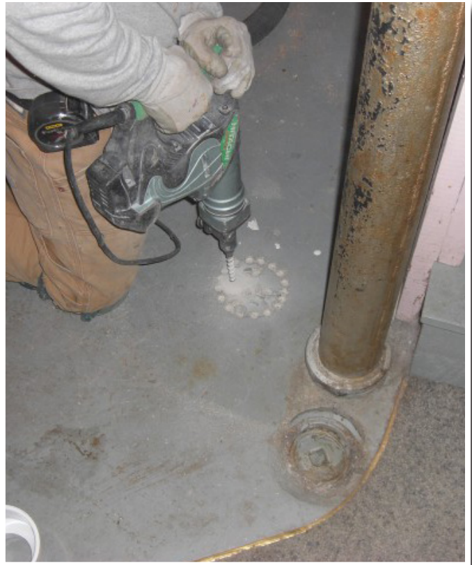
Sub-slab radon system installation.
